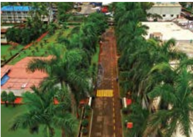
Sudarshan Chemical Industries, Plant View
